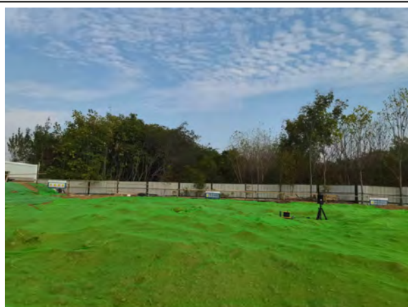
临时施工围挡及裸土覆盖防尘网
